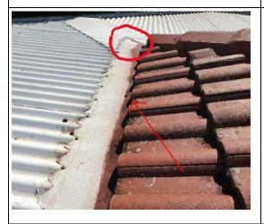
The metal apron flashing to the pergola area where it meets the roof tiles, has been carried out to a tradesman like standard and is in a good condition.
