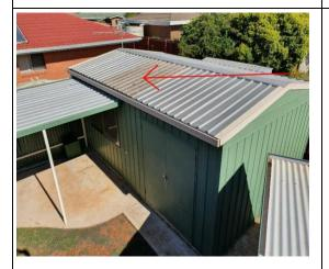
The external of the shed is in a good condition. The Alsynite roof sheeting is starting to show signs of aging. Eventually these alsynite sheets will need to be replaced.
