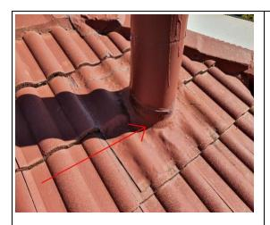
The lead flashing to the fireplace flue in good condition. There was no splitting to the lead flashing.
