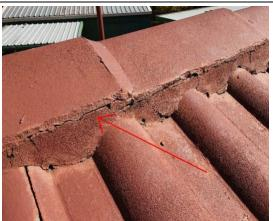
Generally the roof tiles are in a good and sound condition. There are several areas that have hairline cracking to the mortar joints on the ridge capping.
