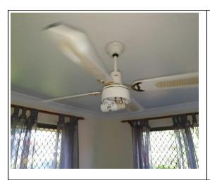
The light shade to the ceiling fan in the main bedroom is not installed.
