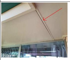
The fibro on the soffit at the front of the house is coming out of the joiner strip.
