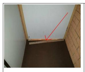
The weather seal to the back door has fallen off and will need to be reinstalled.
