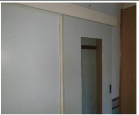
The sliding door in the garage has come off the track and would not open. Seek further advice from a carpenter.
