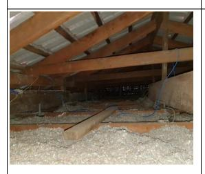
The roof framing appears to be in a good condition and structurally sound for the age of the building. There were no significant structural issues noticed at the time of the inspection.
