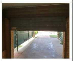
The roller door was working at the time of the inspection. The door is tending to close by itself when not fully opened. It would be recommended to have this door adjusted.
