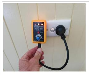
Several of the PowerPoints were tested at the time of the inspection. There does not appear to be any issues or faults with the Power Points.
