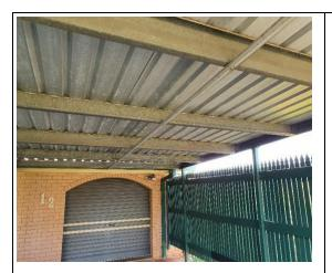
The carport at the front of the building appears to be structurally sound and in a good condition. There is some minor wear and tear to the paintwork that is to be expected for the age of the building.
