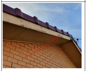
The barge boards at the front of the house are going to require painting to maintain the appearance and prevent dry rot occurring to the timber over time.
