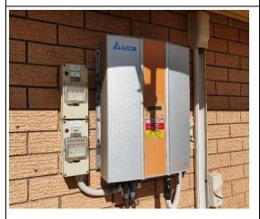
The inverter for the solar panels was working at the time of the inspection. The unit is currently producing electricity back into the grid. There does not appear to be any issues with this unit.
