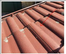
There is a hairline crack to a roof tile on the left-hand side of the building. It would be recommended to have this tile replaced or initially apply Silicon to this crack.
