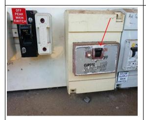
The safety switch in the metre box was working at the time of the inspection and is compliant. This switch is showing signs of aging. It would be suggested to have this safety switch replaced in the near future to maintain the integrity and safety reliability.
