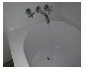
The water was flowing away when tested. There does not appear to be any blockages to the drainpipes.
