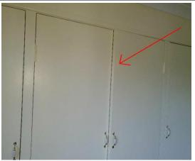
The cupboard doors in the main bedroom are out of alignment and will need to be adjusted.
