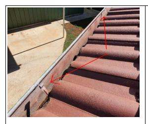
Several of the gutter brackets have popped out of the gutter. These brackets will need to be adjusted. Seek further advice from a roof plumbing contractor or Handyman.
