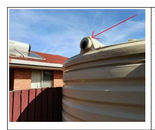
The overflow pipe on the rainwater tank has not been installed. It would be recommended to have a Plumber install this downpipe on the tank and the water diverted away from the building.
